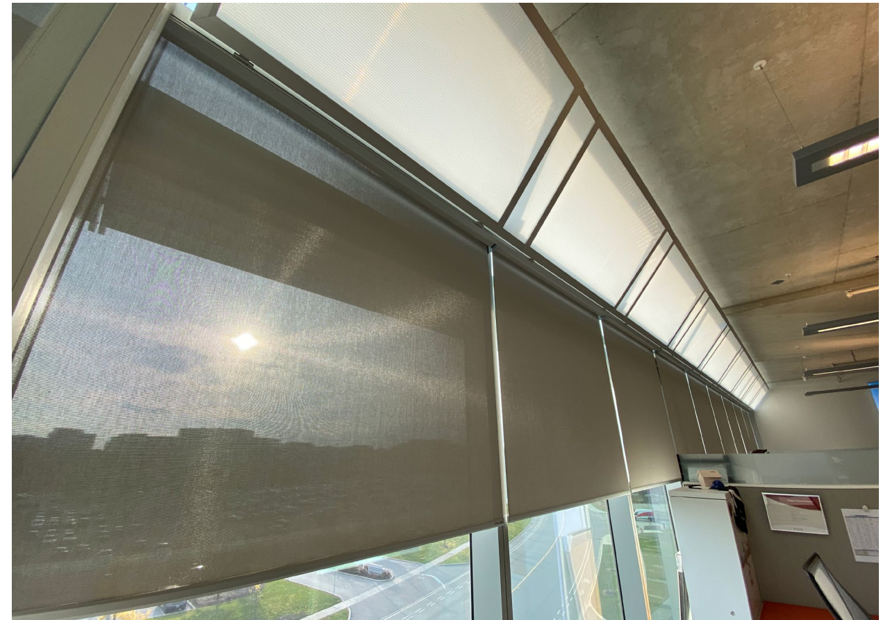
At Mississauga's 5015 Spectrum Way, rooftop sensors follow the angle and position of the sun—day by day, season by season—and direct an integrated system of Legrand lightshelves and shades to adjust for optimal interior daylighting.
